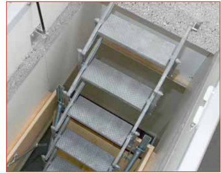
» Extension of scissor stairs (plenum 3)
