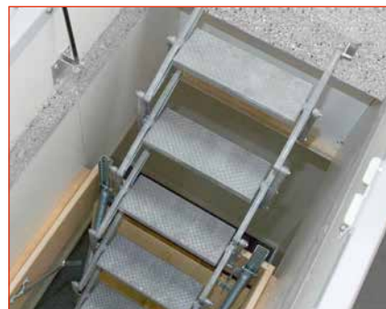
» Extension of scissor stairs (plenum 3)
